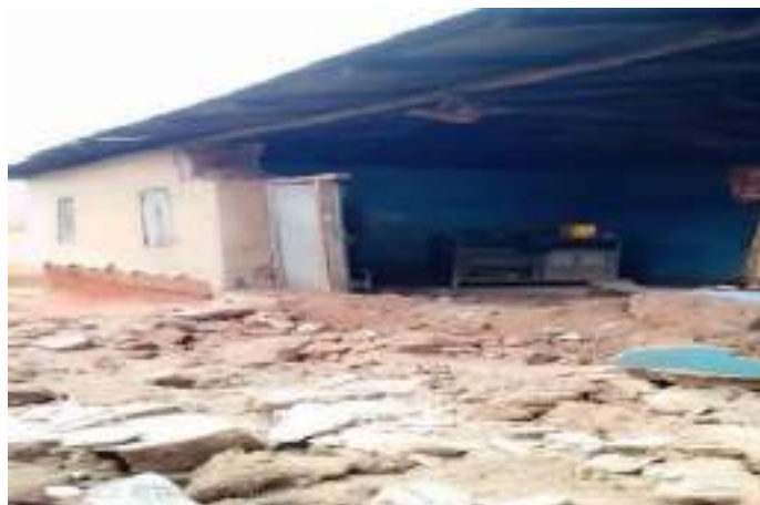
Side wall of a building collapsed due to windstorm
